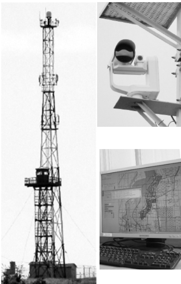
Figure 1 – Example of OSS tower and devices
