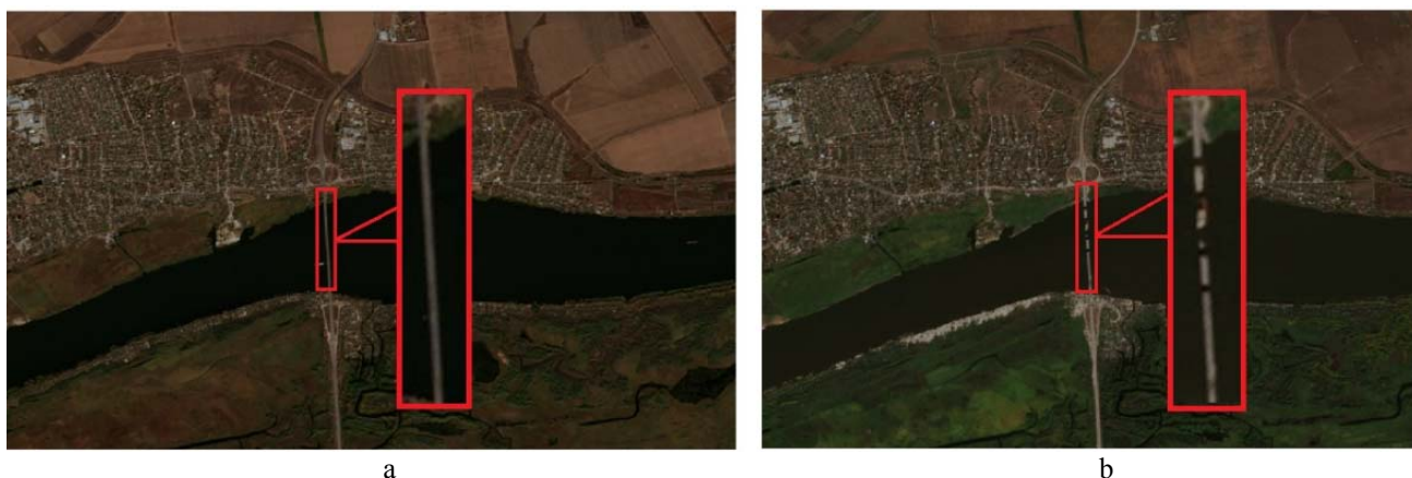
Figure 2 – Multi-temporal Sentinel-2 images of the Antonivsky Bridge: a – 2021 before destruction; b – 2023 after destruction
