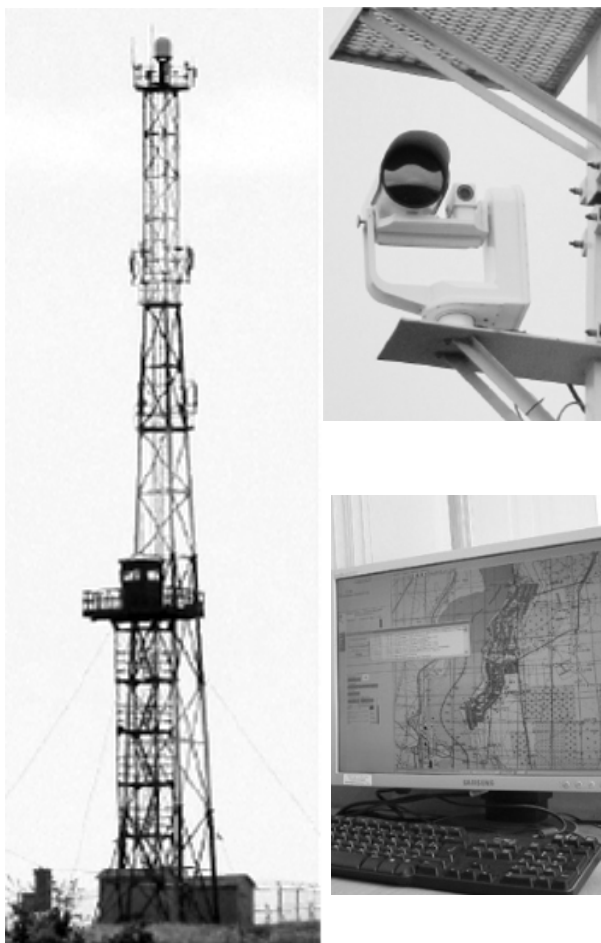
Figure 1 – Example of OSS tower and devices
